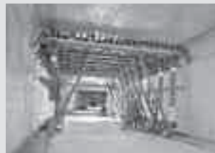
Tunnel Formwork
