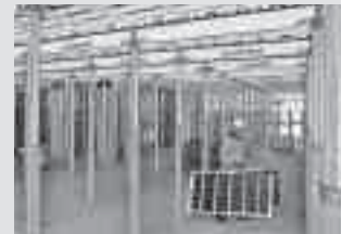
Slab Formwork
