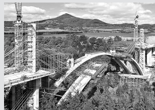
Bridge formwork
