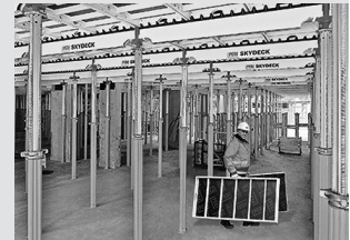
Slab formwork
