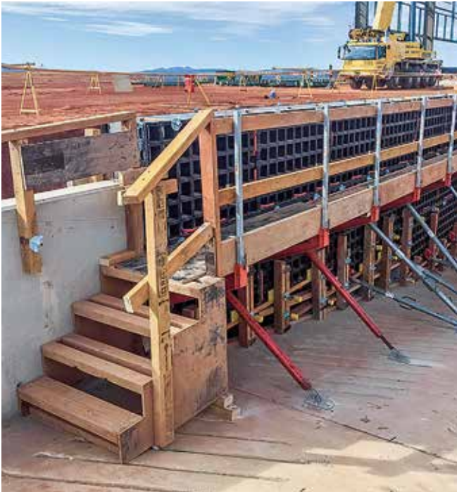
Using the DUO system resulted in a considerable increase in efficiency on the construction site.
