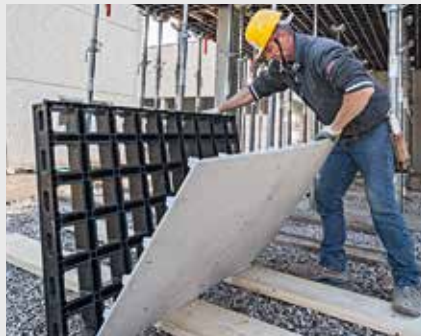
2. Removing the damaged formlining
