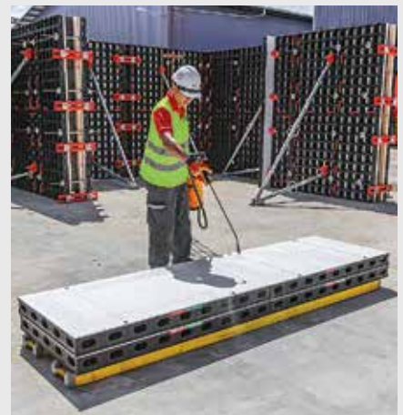
The release agent PERI Plasto Clean can be applied easily using the release agent pressure sprayer.
