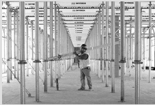
Slab Formwork
